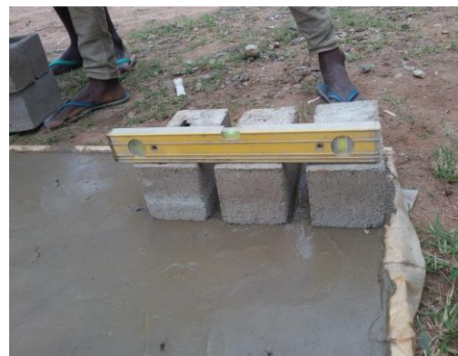
Plate 2.5: Capping Blocks with Cement Mortar
